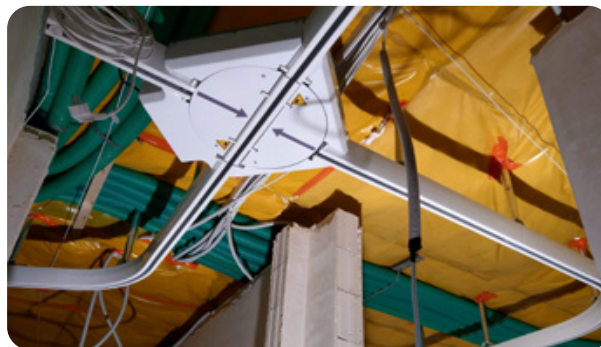
Hook type trolley HOOK-L
